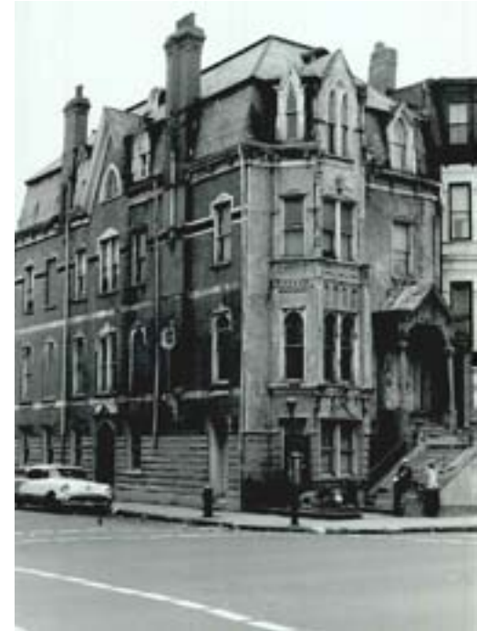
511 Columbus Avenue, ca. 1964 (Photograph by James Kermegis for the Boston Redevelopment Authority, Courtesy of the Boston Landmarks Commission)
