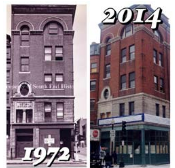
407 Shawmut Ave (Royal Arcanum Building) Then: Boarded up Salvation Army Harbor Light (1972) Now: Construction on "The Royal" condominiums (2014)
