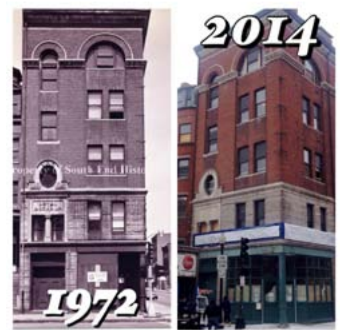
407 Shawmut Ave (Royal Arcanum Building) Then: Boarded up Salvation Army Harbor Light (1972) Now: Construction on "The Royal" condominiums (2014)
