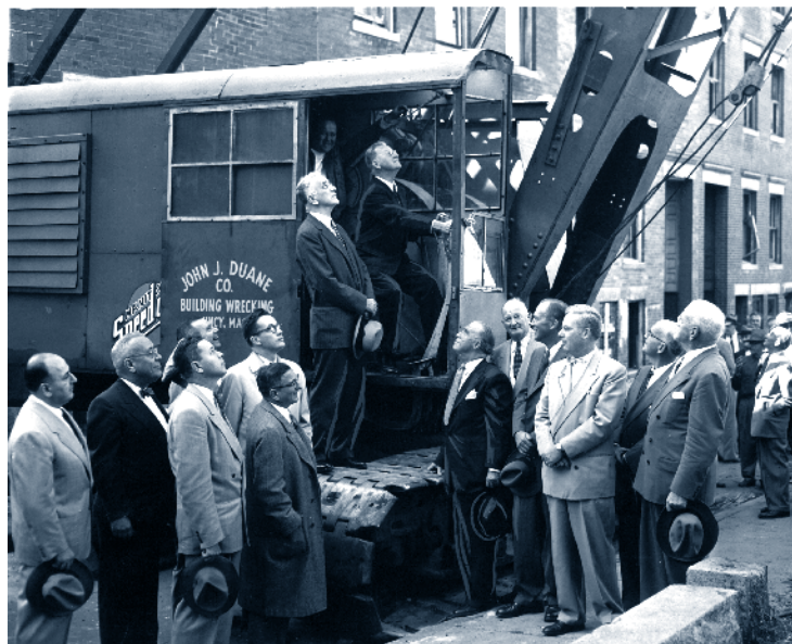
Mayor John B. Hynes operates controls of a wrecking crane on Seneca Street, September 23, 1955. Courtesy of Boston Public Library, Print Department.
